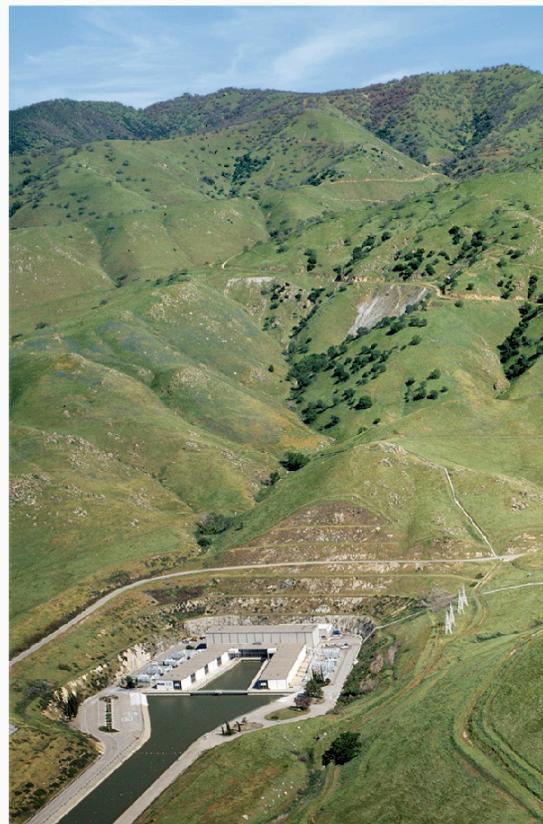
A. D. Edmonston Pumping Plant.
