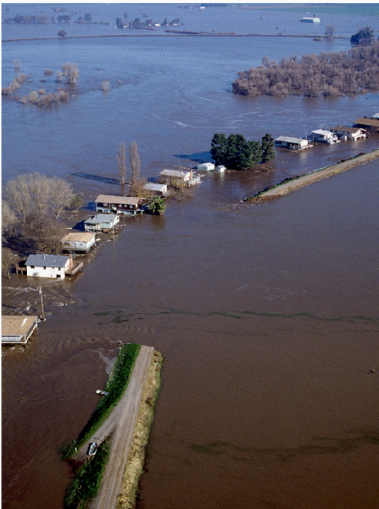
Delta levees are prone to failure, increasing risks to State water supplies.
