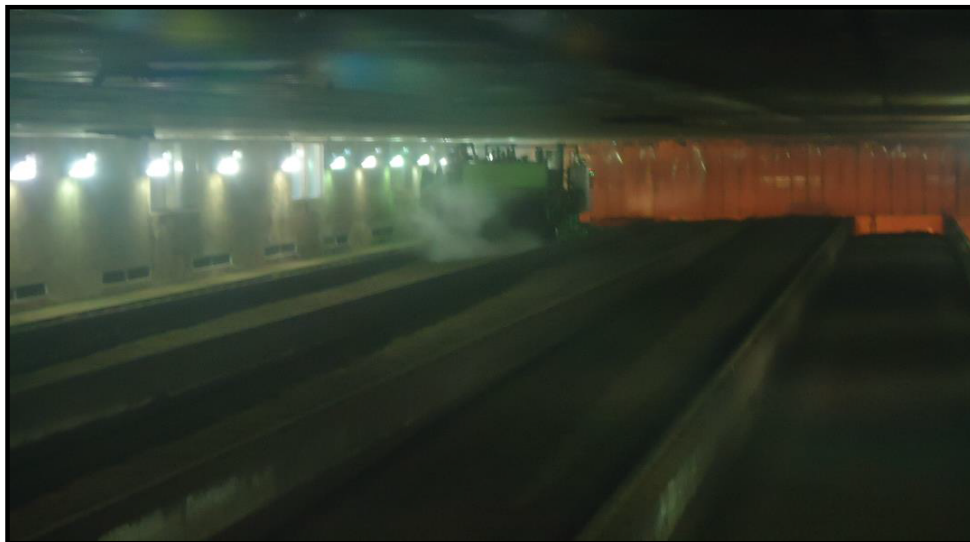
Las Virgenes MWD's indoor composting facility
