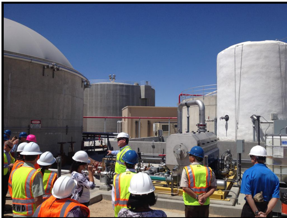
Anaerobic Digesters at Victor Valley WRA's WRP-San Bernardino County
