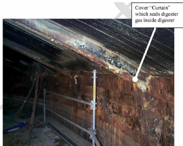
Figure 1 – Digester No 2 Cover Corrosion, Especially on “Curtain”
