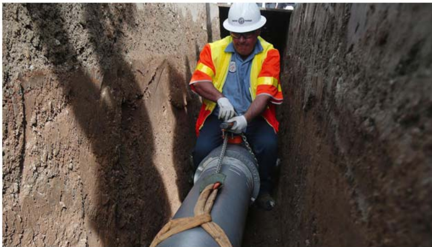
Los Angeles DWP crews replace a water main
