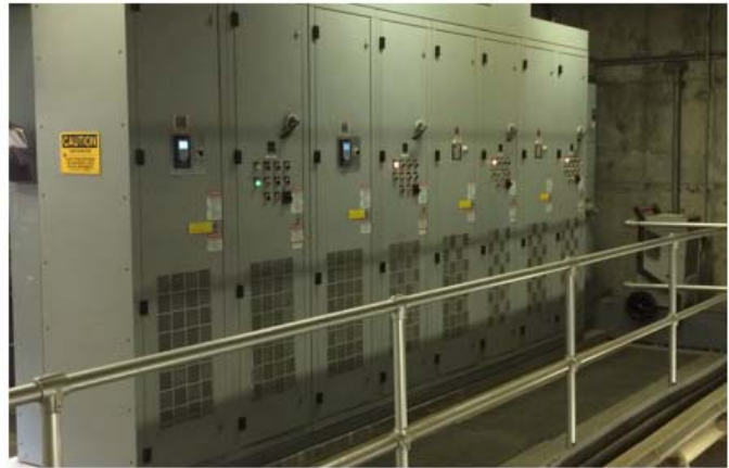
Indoor electrical equipment at Lift Station No. 1.
