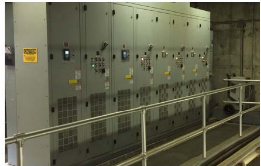
Indoor electrical equipment at Lift Station No. 1.
