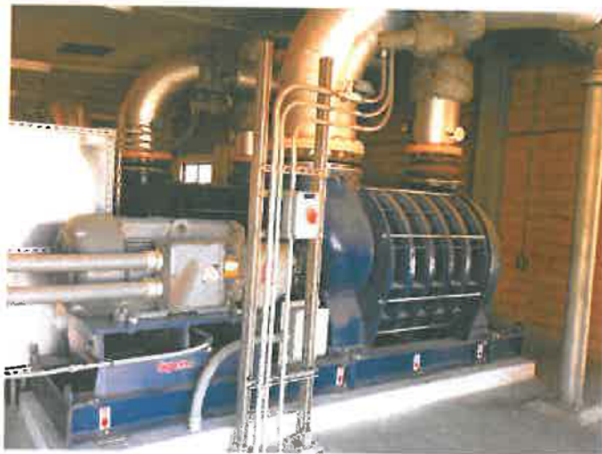
Figure 3: Blowers for the IFAS Process
