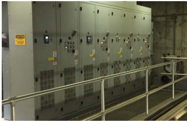
Indoor electrical equipment at Lift Station No. 1.
