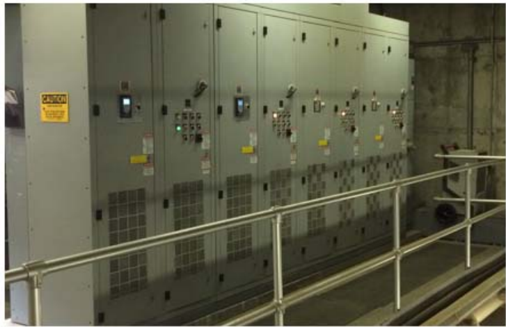
Indoor electrical equipment at Lift Station No. 1.
