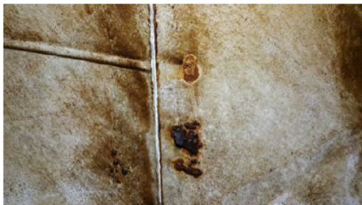
Spot of corrosion on the interior of the pipe
