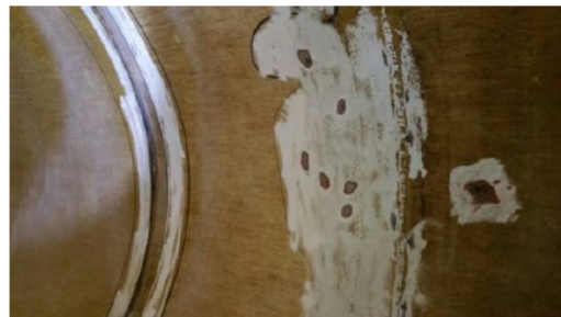
Surface preparation on the interior of the pipe
