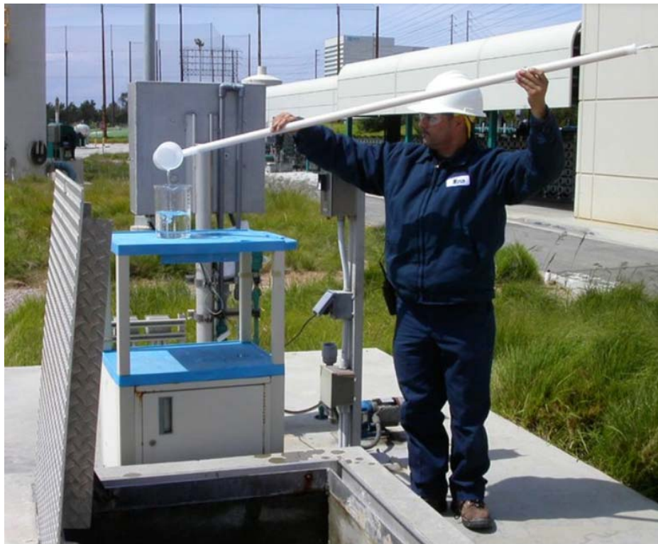
An engineer samples recycled water at Delta Diablo Sanitation District in Oakley, Calif. The district has applied for a $4.4 million loan from the Clean Water State Revolving Fund to build storage tanks for recycled water. Delta Diablo Sanitation District
