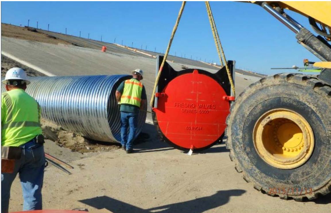
Workers install pipes and valves as part of the EchoWater Project, an effort by the Sacramento Regional County Sanitation District to clean up the effluent it discharges to the Sacramento River. Some of this effluent will be diverted to a new network of distribution pipes that will irrigate farmland. (Sacramento Regional County Sanitation District)
