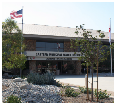
Eastern Municipal Water District's headquarters is home base for leak detection and water conservation in Riverside County, California.
