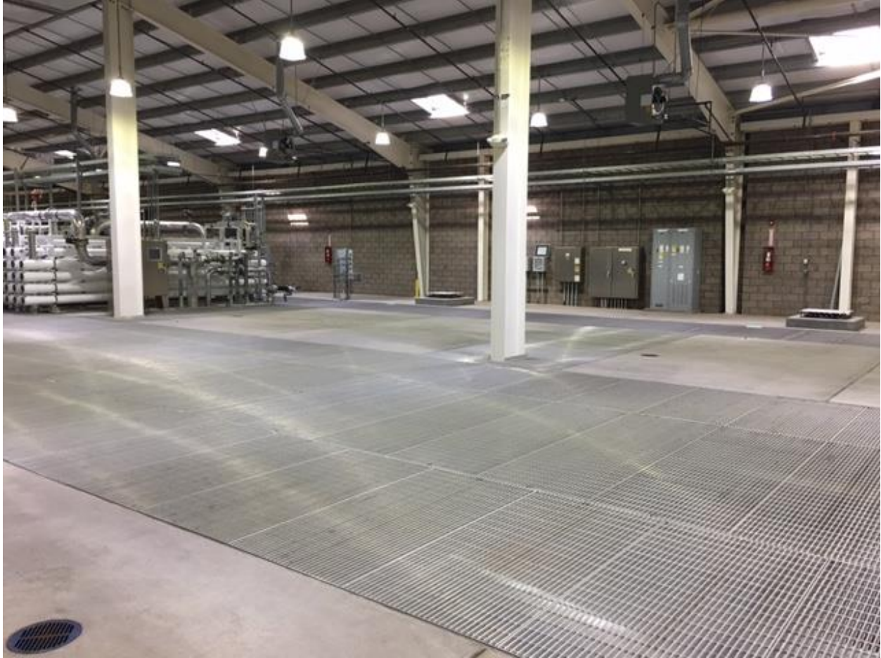
Available space for two new 3.0 mgd NF treatment trains at the Yucaipa Valley Regional Water Filtration Facility.
