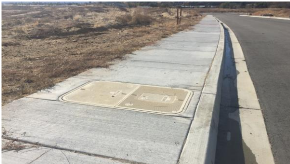
YVWD standard meter boxes for dual-plumbed communities.
