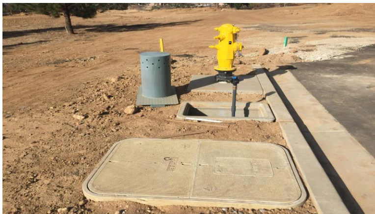
YVWD meter box without a sidewalk for a large-lot, rural application.
