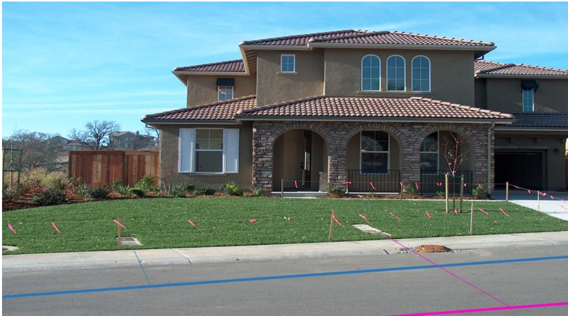
Meter boxes from a dual-plumbed community in northern California.
