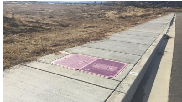
YVWD standard meter boxes for dual-plumbed communities.
