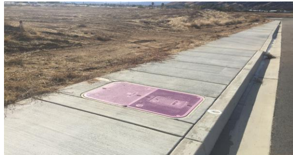
YVWD standard meter boxes for dual-plumbed communities.
