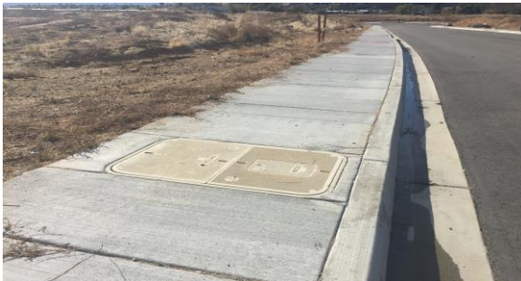
YVWD standard meter boxes for dual-plumbed communities.
