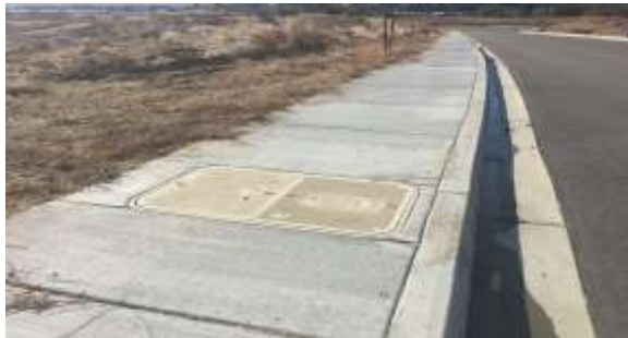
YVWD standard meter boxes for dual-plumbed communities.
