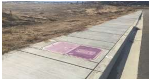
YVWD standard meter boxes for dual-plumbed communities.
