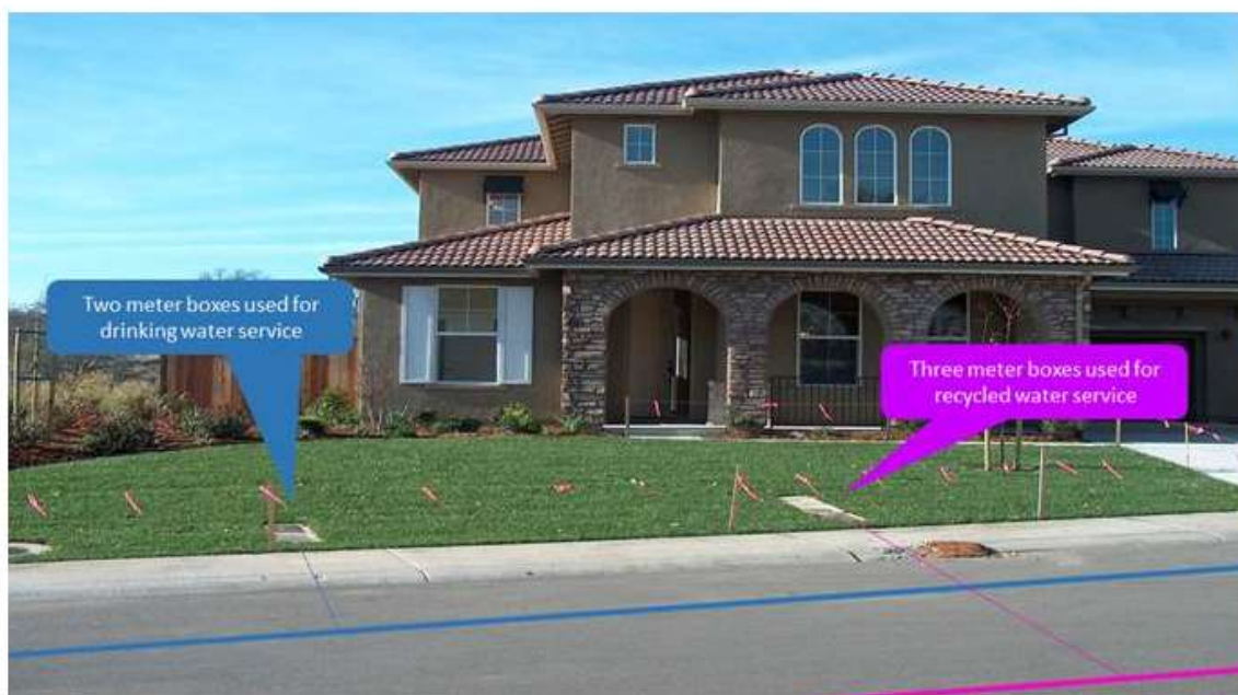
Figure 1 - El Dorado Irrigation District Dual-Plumbed Installation
