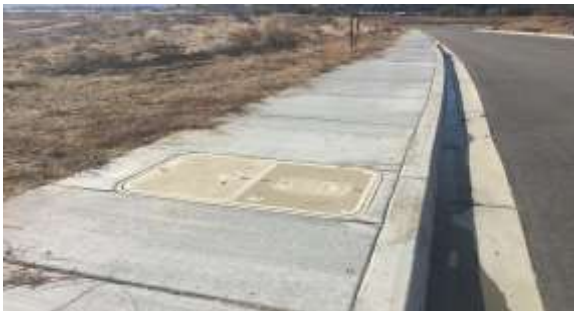
YVWD standard meter boxes for dual-plumbed communities.
