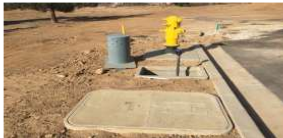
YVWD meter box without a sidewalk for a large-lot, rural application.
