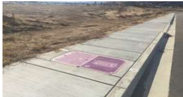
YVWD standard meter boxes for dual-plumbed communities.
