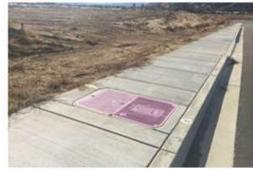
Figure 2 - YVWD Standard Meter Boxes for Dual-Plumbed Communities
