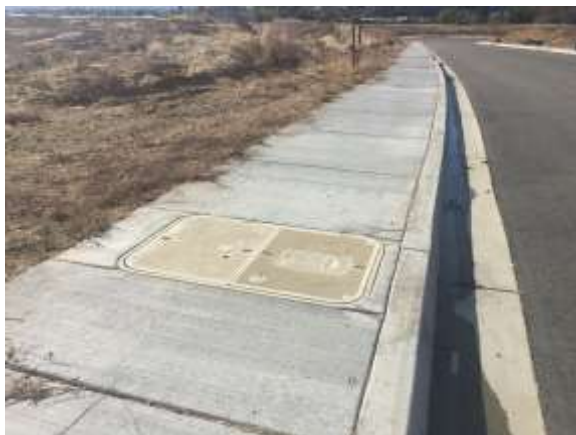
YVWD standard meter boxes for dual-plumbed communities.
