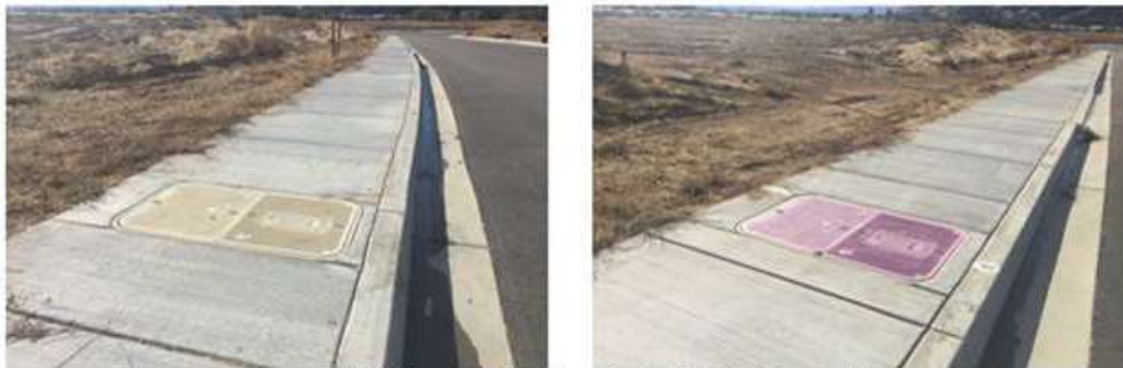
Figure 2 - YVWD Standard Meter Boxes for Dual-Plumbed Communities
