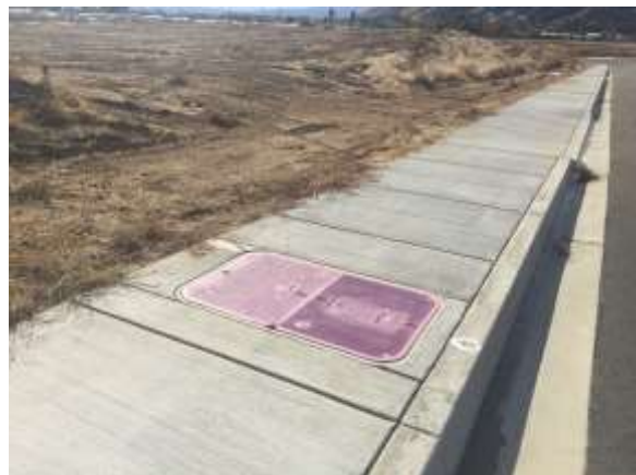
YVWD standard meter boxes for dual-plumbed communities.
