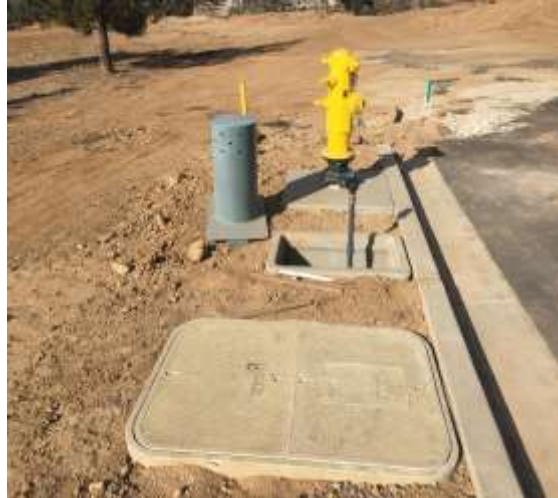
YVWD meter box without a sidewalk for a large-lot, rural application.
