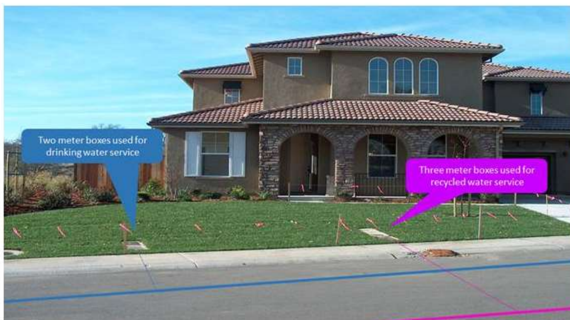
Figure 1 - El Dorado Irrigation District Dual-Plumbed Installation
