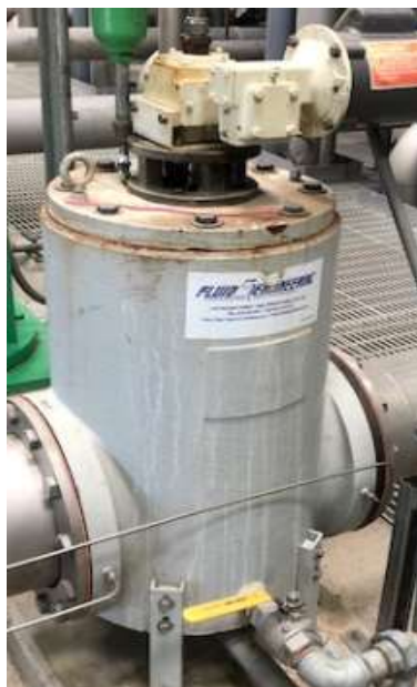
Existing strainer upstream of microfiltration membranes
