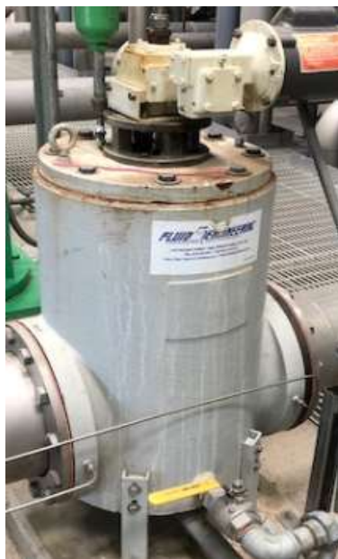
Existing strainer upstream of microfiltration membranes
