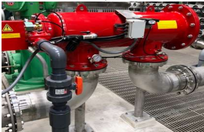
New strainer upstream of future ultrafiltration membranes
