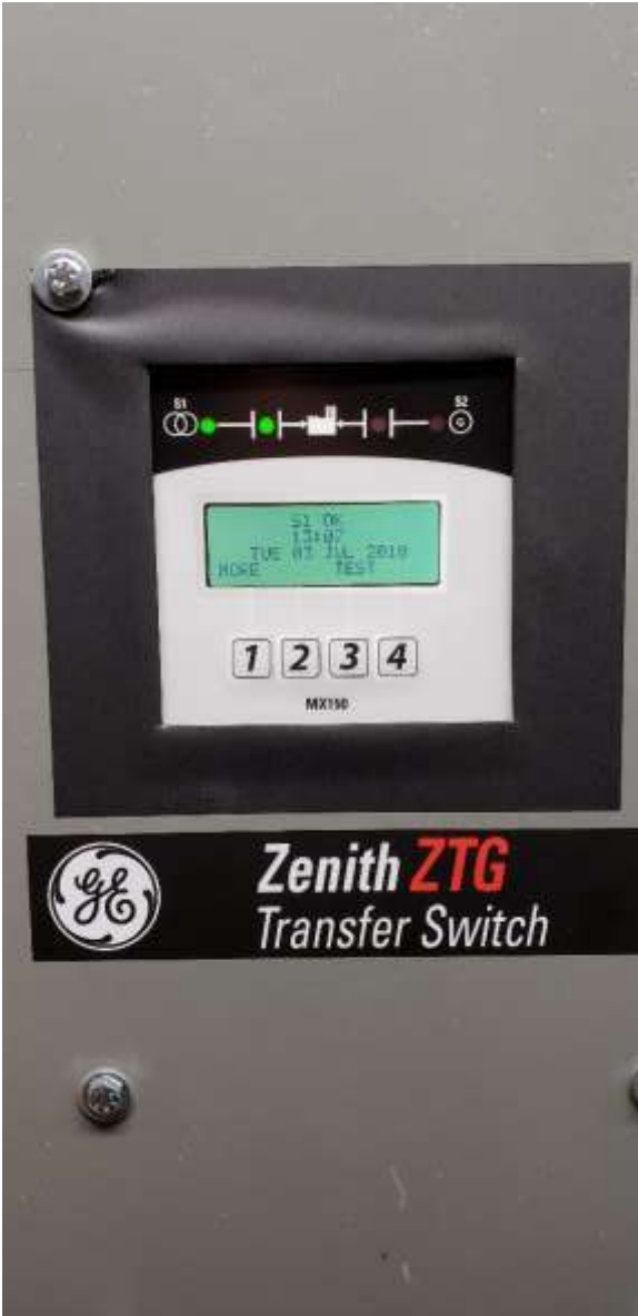
Exterior Mounted ATS Digital Controls
