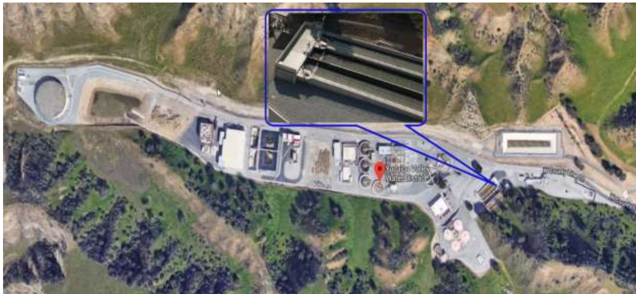
Overview of Wastewater Plant with Primary Clarifier Building Location
