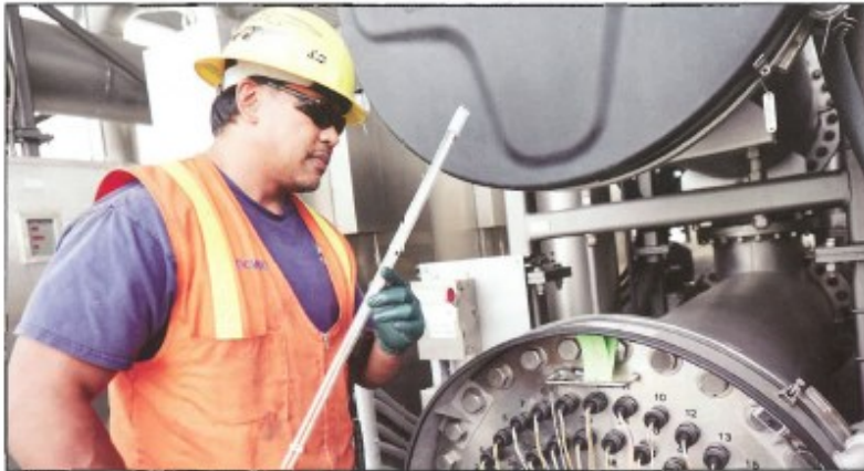
Joseph Flint, lead maintenance technician of Orange County Water District, checks UV lights in the treatment facilities of the Groundwater Replenishment System.
