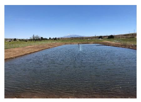
On April 20, 2019, the initial test was stopped to re-evaluate the project due to slow infiltration. The District staff drained the basin, tested the soils in the basin, and removed additional soil from the basin to reach a more permeable layer of soil. Following the modifications to the basin, the District staff and Geoscience restarted the infiltration investigation.
