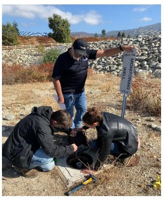
Since groundwater recharge activity is currently taking place at Wilson Creek and Oak Glen Basins, it is advantageous to install monitoring equipment at both locations. Geoscience will assist District staff with the water level and conductivity transducer installation. This will also give District staff a training opportunity of transducer installation, allowing for future installation and data collection to be performed by District staff members.
