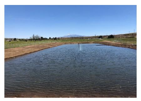
On April 20, 2019, the initial test was stopped to re-evaluate the project due to slow infiltration. The District staff drained the basin, tested the soils in the basin, and removed additional soil from the basin to reach a more permeable layer of soil. Following the modifications to the basin, the District staff and Geoscience restarted the infiltration investigation.
