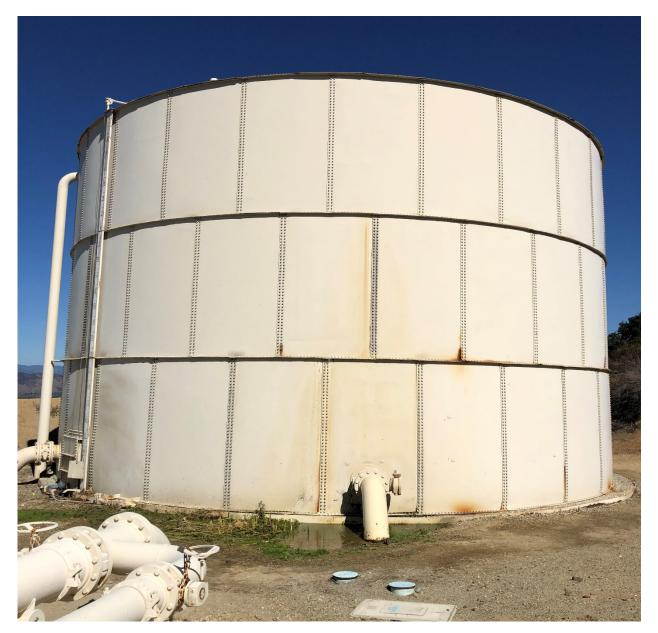
The proposed project would require a temporary storage solution during the demolition and construction of the new tank. If the District staff receives authorization to proceed with this project at the October 15, 2019 board meeting, a new tank can be operational by June 2020. With the deteriorating condition of the existing tank, the timing of the installation of the temporary tank system should be considered a priority.
