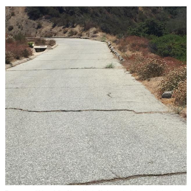
The access road (pictured above) is used by the District to maintain the reservoir site as well as by the property owner of the adjacent parcel and will be paved over the trench after the conduit is installed. The final topcoat slurry seal will be applied over the entire road surface once the all work has been completed as a part of a separate paving contract. The preliminary construction drawings have been completed which will be the basis of the construction contract.
