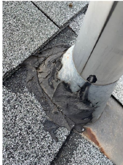
Picture 2: Penetration mastic sampled from the roof
