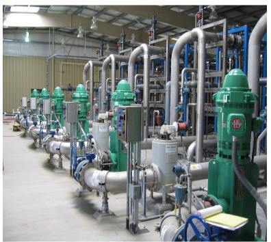
The proposed Forsta auto strainer equipment would provide the microfiltration membranes with high quality filter feed water with a 300-micron screen rating. While the Forsta strainers have a
