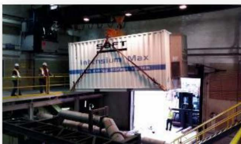
Ameresco installed a 500kW/580kWh SAFT Lithium Ion BESS at the Portsmouth Naval Shipyard in 2015
