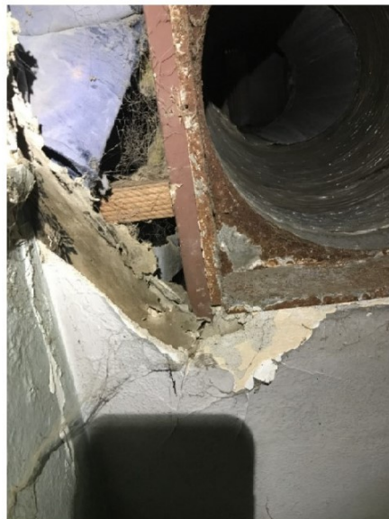
Picture 11: Plaster sampled was found to not contain asbestos
