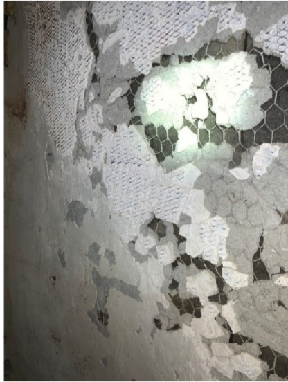
Picture 5: Exterior stucco was found to not contain asbestos
