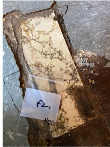
Picture 2: Asbestos-containing sheet flooring
