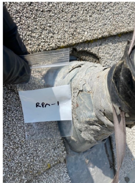
Picture 3: Asbestos-containing roofing penetration mastic around the ducts
