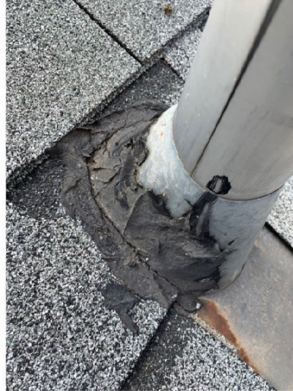
Picture 2: Penetration mastic sampled from the roof
