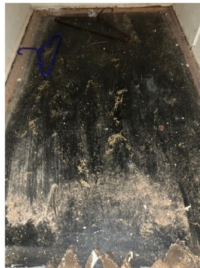
Picture 4: Black flooring sampled in closet was found to not contain asbestos
