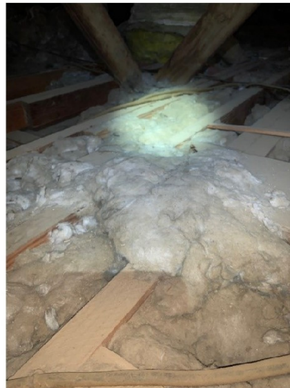
Picture 4: Insulation was found to not contain asbestos
