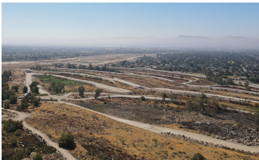
The Waterman and Twin Creek Spreading Grounds capture stormwater and recharge State Water Project to the Bunker Hill-A GMZ.
