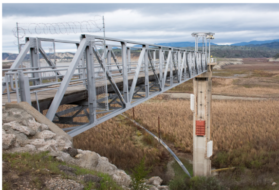
Looking out over Lake Cachuma at the intake tower that feeds water into the distribution system serving the greater Santa Barbara area. The temporary drought emergency pipeline in the lower foreground extends to a barge-mounted pumping plant in the reservoir.
