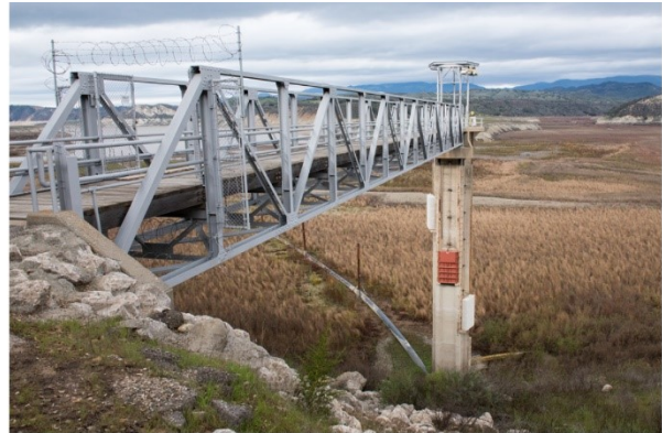
A dry Lake Cachuma in February 2017. The temporary pipeline seen here entering the inlet tower to the Tecolote Tunnel connected a barge-mounted emergency pumping plant on the lake to the inlet. The dry lakebed illustrates lingering Central Coast drought impacts that were not mitigated by a wet Water Year 2017. It was not until early 2019 that lake levels recovered sufficiently to permit decommissioning of the temporary facilities.
