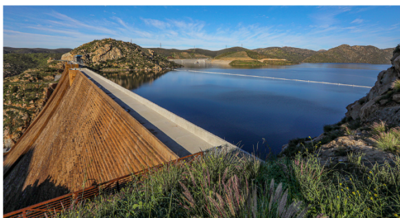
The City of San Diego's San Vicente Dam, constructed in the 1940s, was raised 117 feet as part of San Diego County Water Authority's (SDCWA's) emergency storage project, more than doubling the reservoir's capacity and improving the drought resiliency of a region having relatively little local surface water or groundwater storage capacity. The enlargement was completed in 2014. Photo credit: SDCWA
