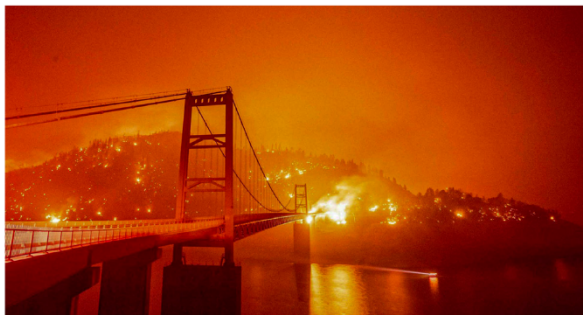
Flames from the Bear Fire in September 2020 burn around Lake Oroville; the Bidwell Bar Bridge is in the foreground. DWR evacuated Hyatt Powerplant as a precautionary measure. The fire destroyed much of the small community of Berry Creek. Similarly, the 2018 Carr Fire burned the area surrounding the U.S. Bureau of Reclamation's Keswick Dam and powerplant, requiring evacuation of plant operators and resulting in boil water advisories for residents served by several small community services districts. Photo credit: Getty Images
