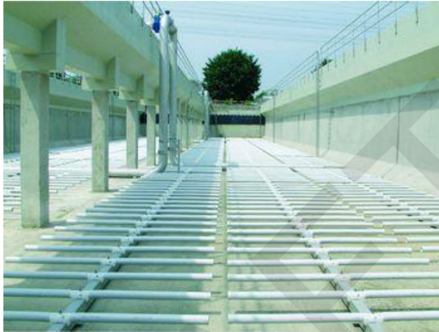
Figure 3-2: OTT Fine Bubble Diffuse Installation
