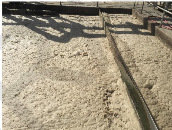
Figure 1-1: Foam in an Aeration Tank
