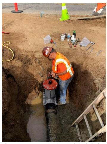
insertion valves that can be installed under live system pressure through a single tap in the host pipe, providing a permanent means of isolation that functions comparably to traditional gate valves.
