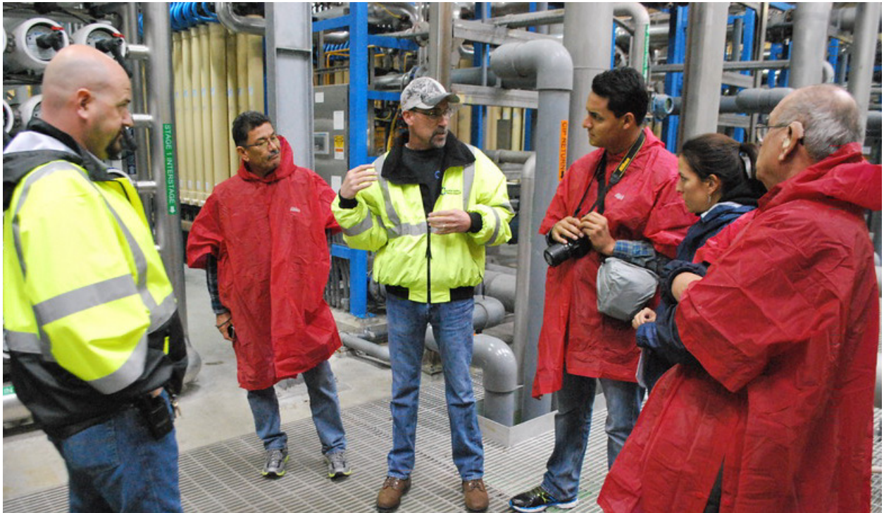
Operations Manager Kevin King discussing the molecular filtration process at the Wochholz Regional Water Recycling Facility.
