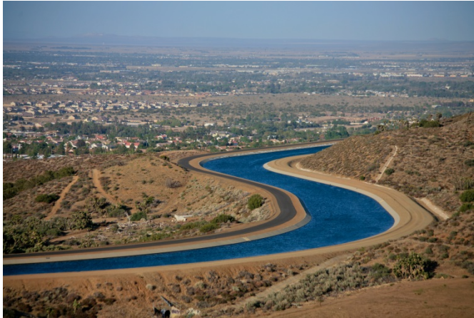
The California Aqueduct delivers imported water to the Upper Santa Ana River Watershed.
