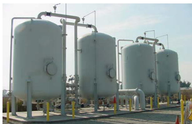
Perchlorate treatment facilities, similar to the West Valley Water District plant above, treat groundwater for use in the Region.
