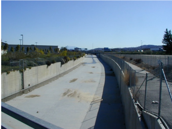
The San Timoteo flood channel is a concrete-lined channel.
