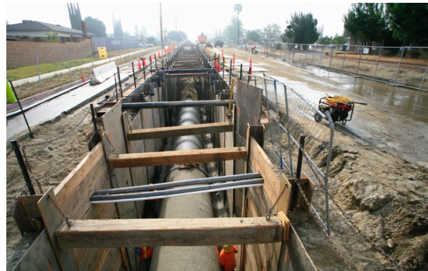
Regional water supply infrastructure delivers local supplies across to the City of Riverside.
