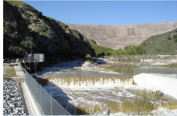
The Cuttle Weir is a concrete and rock diversion structure owned by the San Bernardino Valley Water Conservation District and is used to divert water from the Santa Ana River to the Conservation District's Santa Ana River Spreading Grounds for artificial recharge of the SBBA. The Seven Oaks Dam can be seen in the background.
