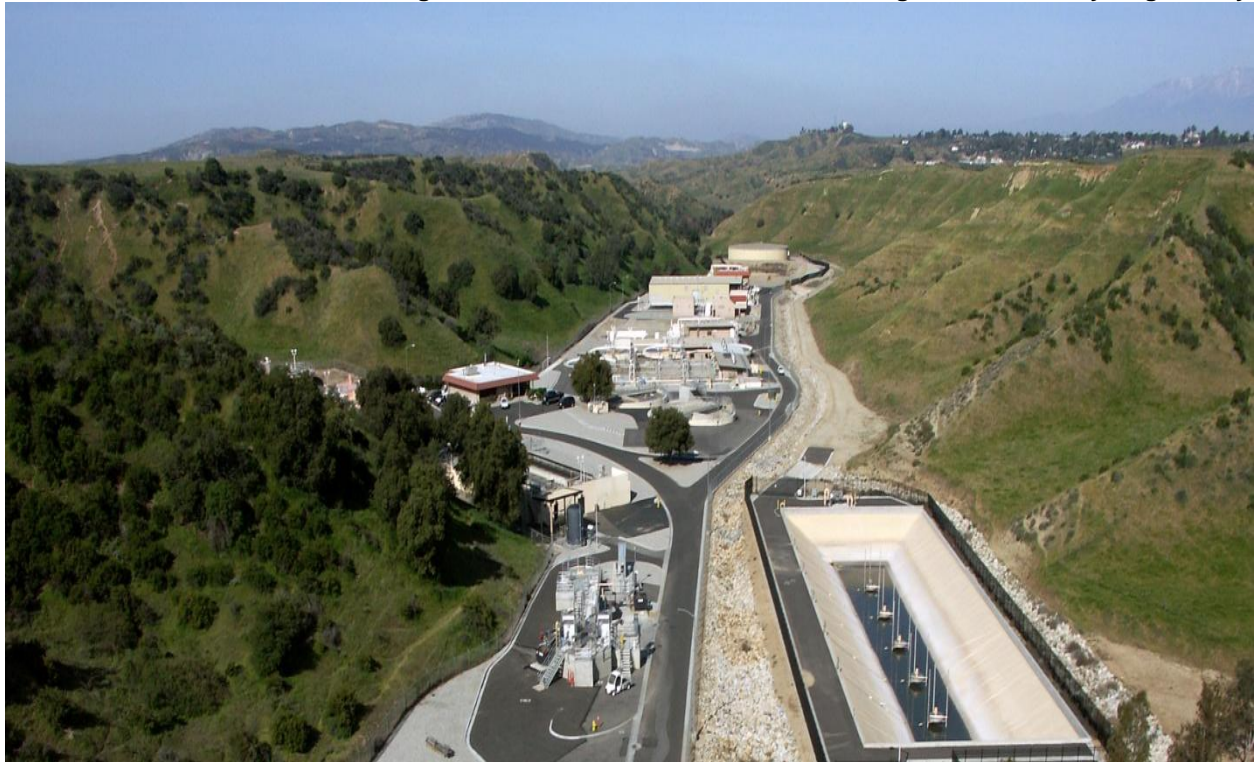
Figure 4-16- Aerial View of the Wochholz Regional Water Recycling Facility
