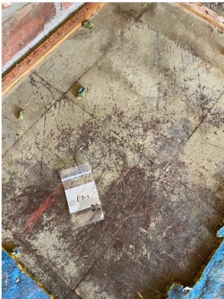
Picture 3: Asbestos-containing brown 9x9 floor tile
