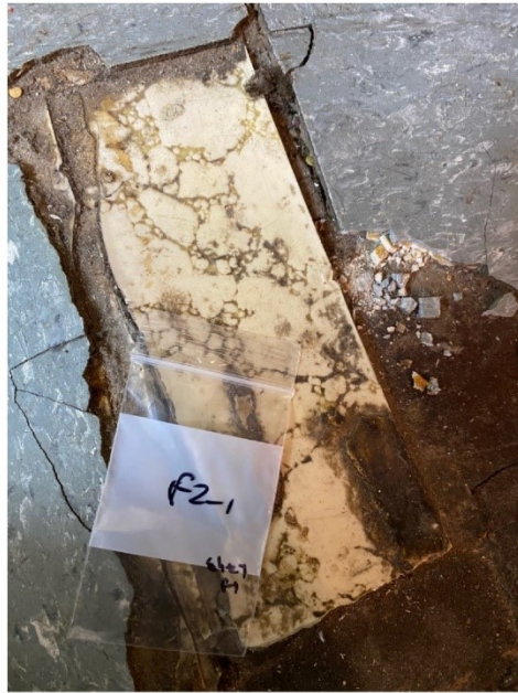
Picture 2: Asbestos-containing sheet flooring
