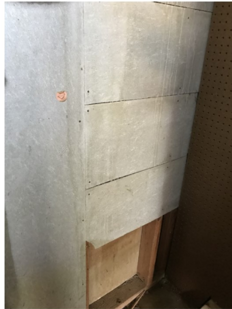
Picture 10: Particle board sampled was found to be ACM
