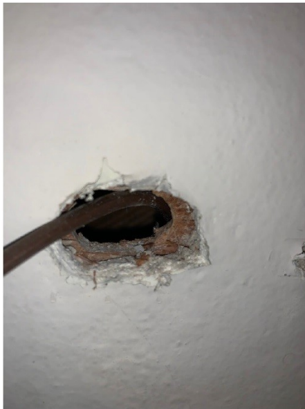
Picture 3: Wall system sampled was found to not contain asbestos
