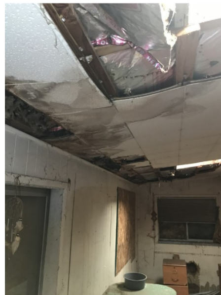
Picture 8: Damaged ceiling tile was found to not contain asbestos
