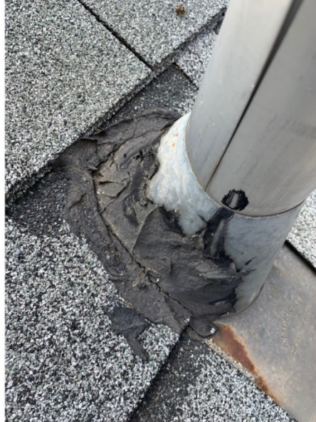
Picture 2: Penetration mastic sampled from the roof
