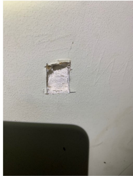
Picture 6: Wall system was found to not contain asbestos
