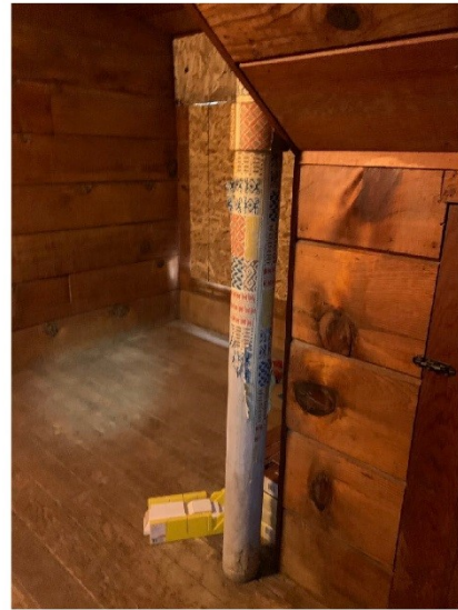
Picture 2: Assumed ACM 6" Transite Pipe running through home
