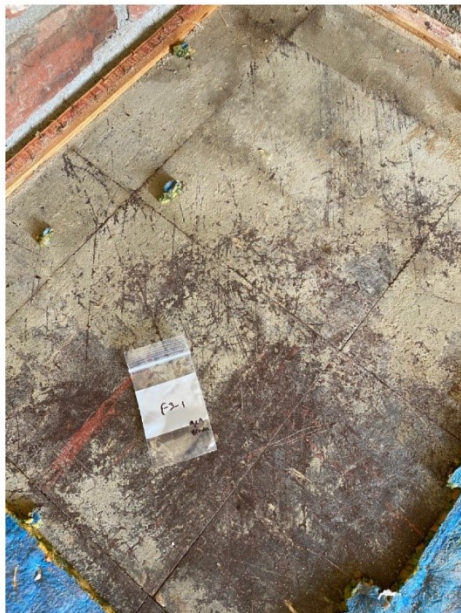
Picture 3: Asbestos-containing brown 9x9 floor tile
