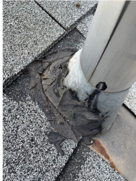
Picture 2: Penetration mastic sampled from the roof
