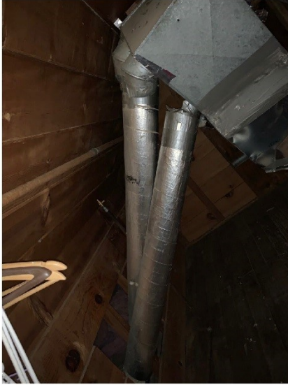
Picture 1: HVAC Duct wrapping in the attic was found to be ACM
