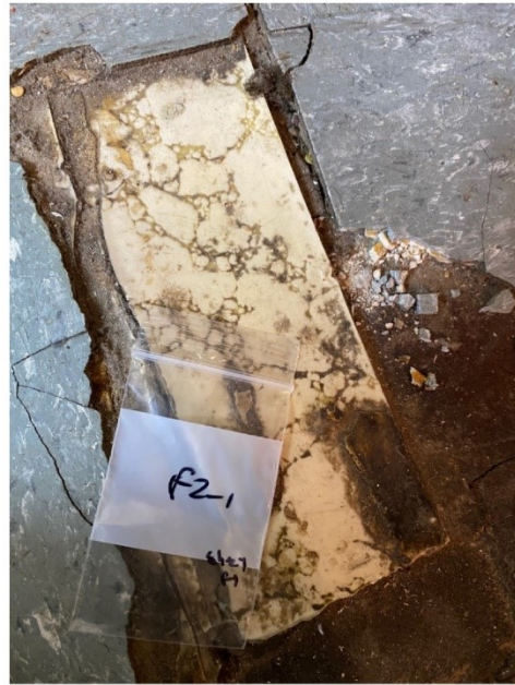
Picture 2: Asbestos-containing sheet flooring
