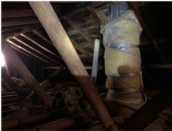
Picture 3: Thermal system insulation around the boiler duct was found to be ACM
