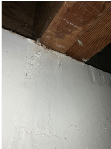
Picture 7: Joint compound was found to not contain asbestos
