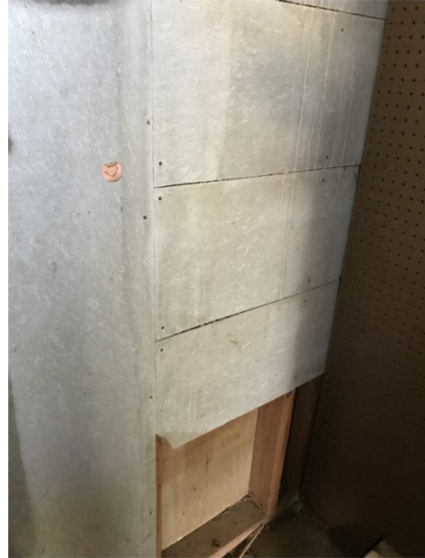
Picture 10: Particle board sampled was found to be ACM
