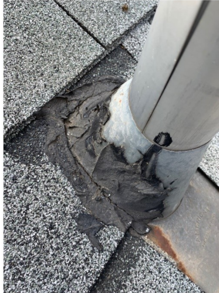
Picture 2: Penetration mastic sampled from the roof
