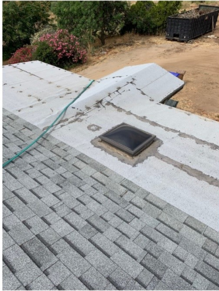
Picture 1: Roofing of the subject property was found to not contain asbestos
