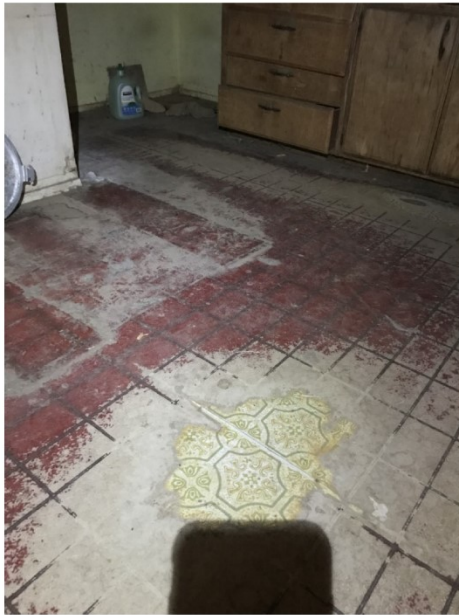
Picture 9: Layered sheet flooring sampled from the kitchen was found to be ACM
