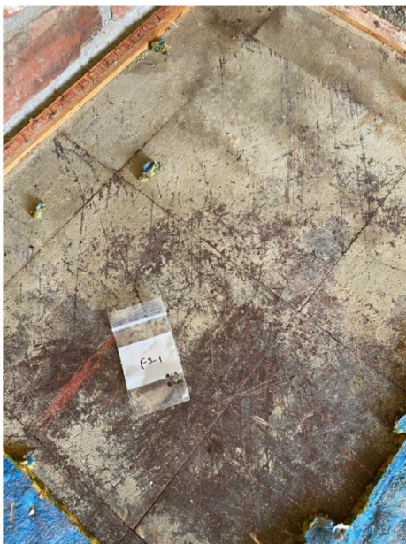
Picture 3: Asbestos-containing brown 9x9 floor tile
