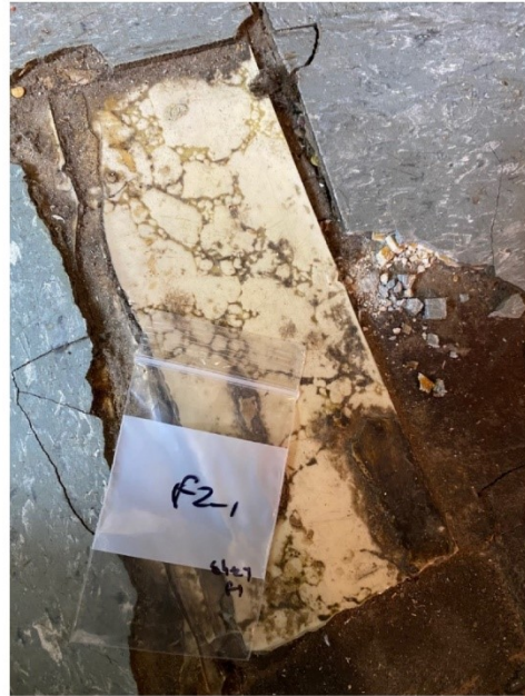
Picture 2: Asbestos-containing sheet flooring
