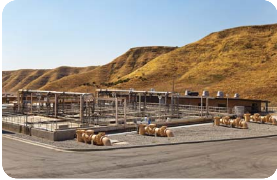
Overview of Wochholz Water Recycling Facility
