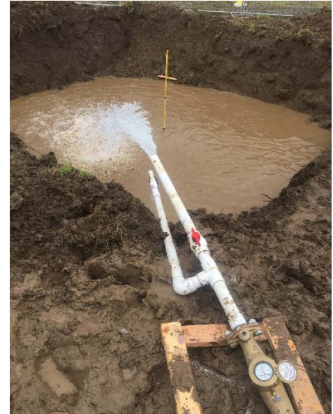
Example: Infiltration Test at Ford Ponds Santa Clara Valley Water District
