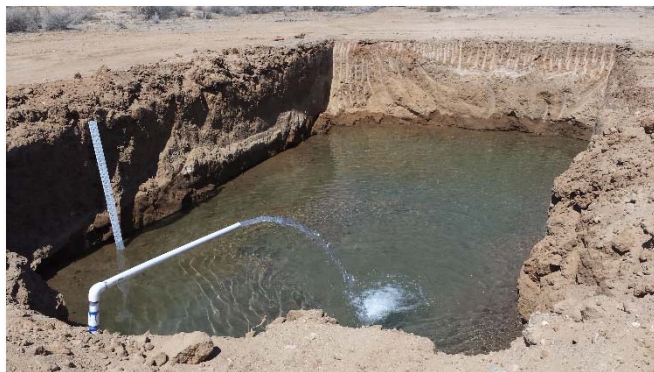
Example: Infiltration Test in Alto Subarea, Mojave Water Agency (manual flow control and water level monitoring)
